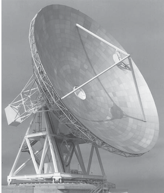
Figure 8.7 Standard-A (C-band 6/4 GHz) 32-m antenna. (Courtesy of TIW Systems, Inc., Sunnydale, CA.)
