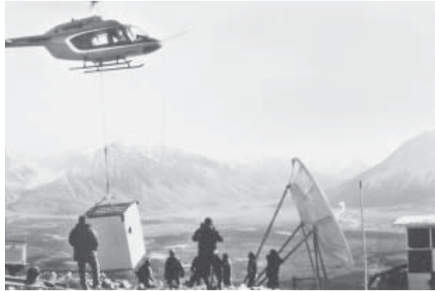
Figure 14.7 Transportable message station. (From Telesat Canada, 1983.)
